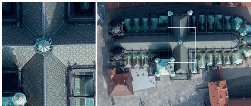
▲ Figure 3, Part of the orthomosaic and detail (left).
