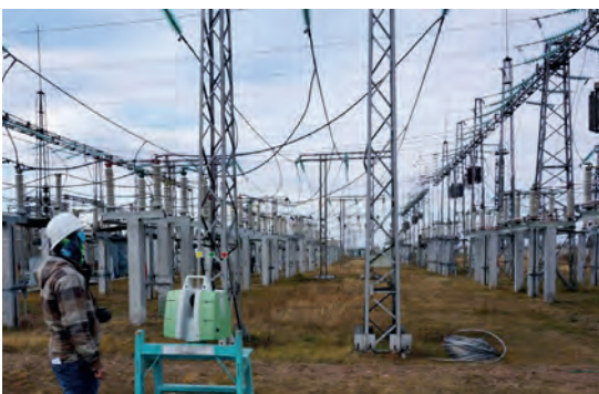
▲ Figure 1, Laser scanning of the power substation.
