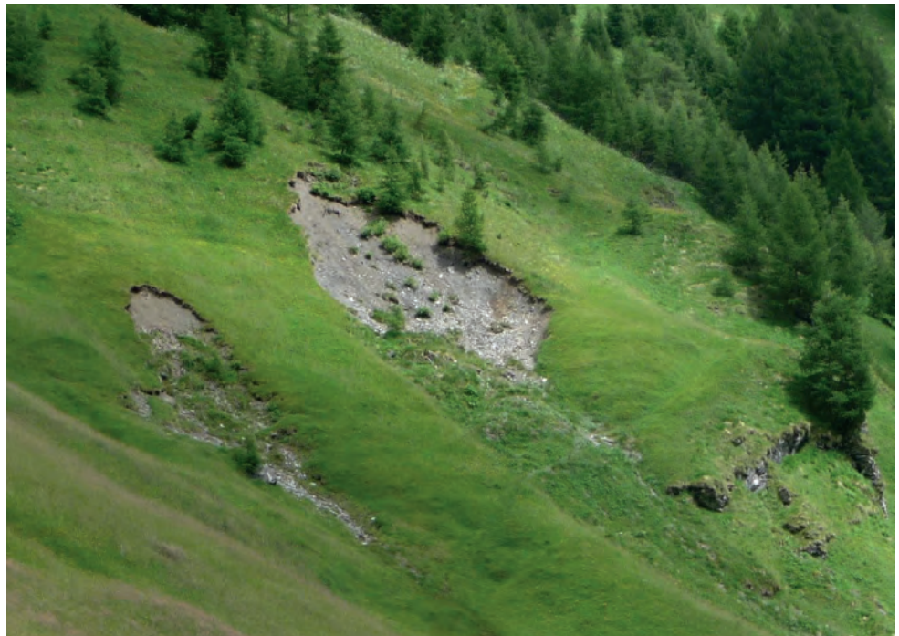
▲ Figure 2: Test site with two shallow landslides.
